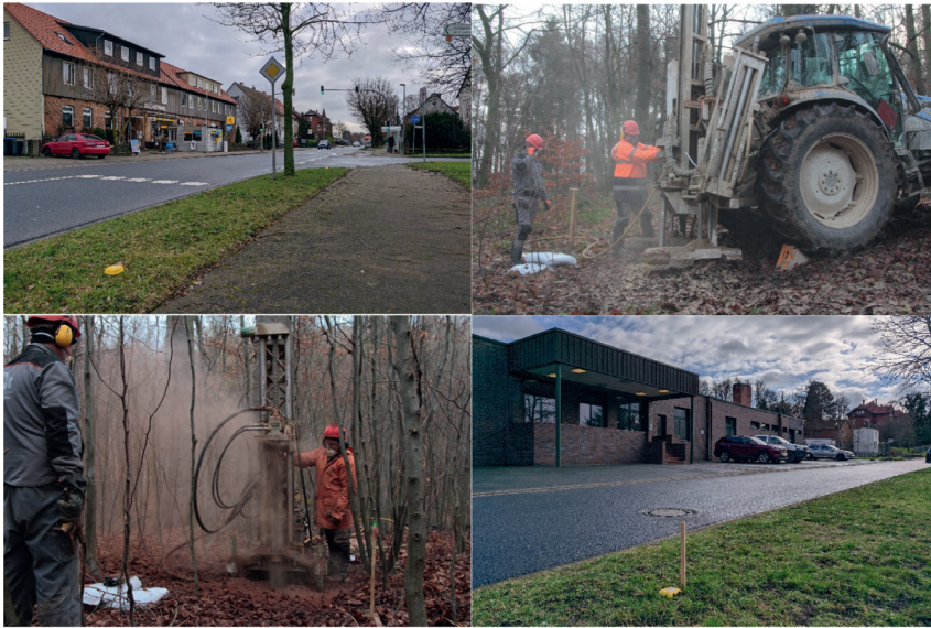
Figure 6 Examples of Quantum nodes layout in urban areas and drilling operation in forest areas.
